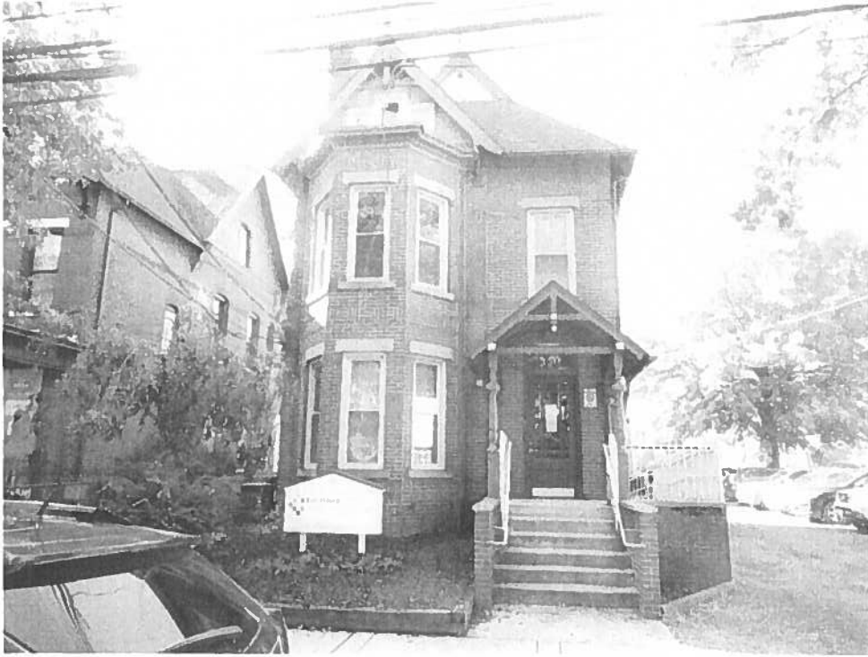
FRONT VIEW OF SUBJECT FACING SOUTHERLY
