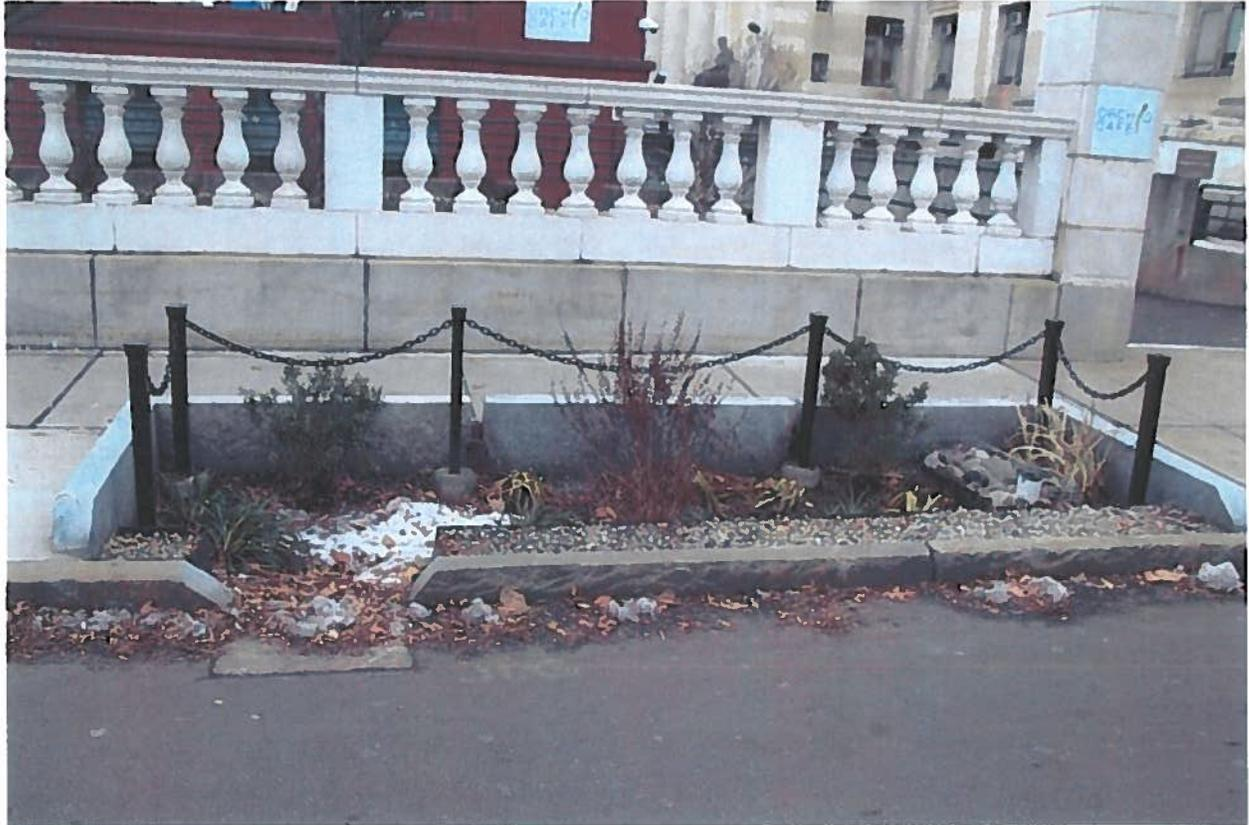
You can't put a bioswale on a hill. And bioswales must leave at least five feet of sidewalk for pedestrian passage. That posed a bit of challenge, in front of the library, with its steps and walls pushing out towards the curb.
