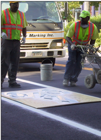
Bike lane installation, New Haven
