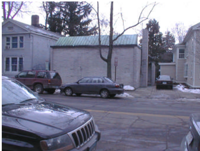
Figure 6.15. Incompatible building forms or street facings.
