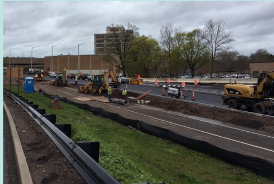
Orange Street Intersection
