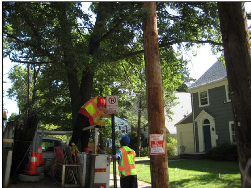
Traffic calming on Vista Terrace.
