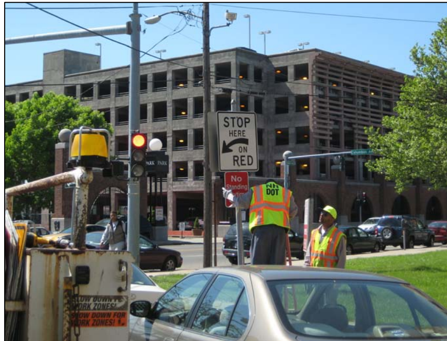
Repair of traffic control signs at Union Station.
