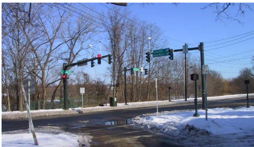
New signals are equipped with video detection and pedestrian enhancements.
