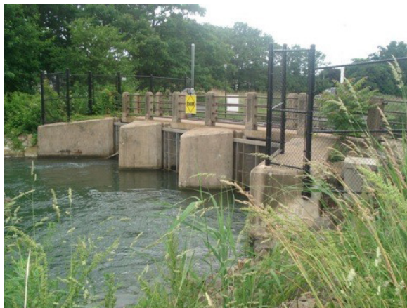
Floodgates installed at Dean Street in Morris Cove neighborhood.
