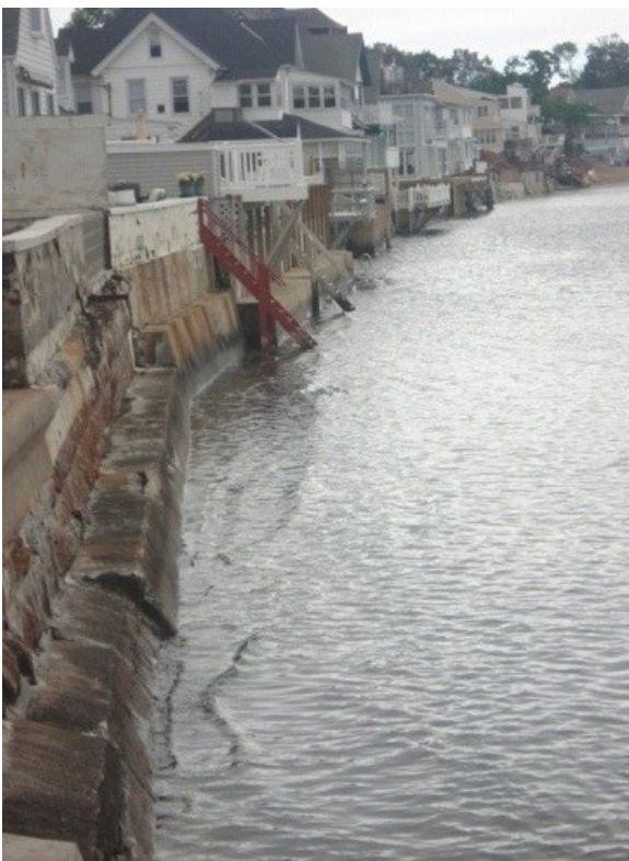
View of properties at risk at Pardee seawall in Morris Cove neighborhood.
