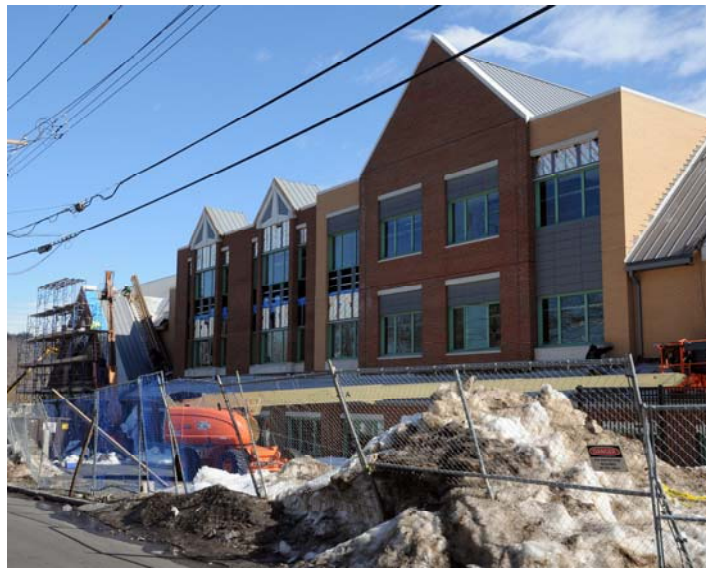
Ongoing construction of the Davis Street School.
