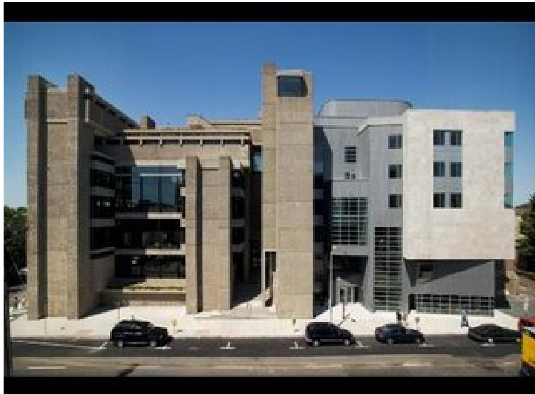
Yale School of Architecture, left, a Brutalist masterpiece, alongside the new Loria Art History building.
