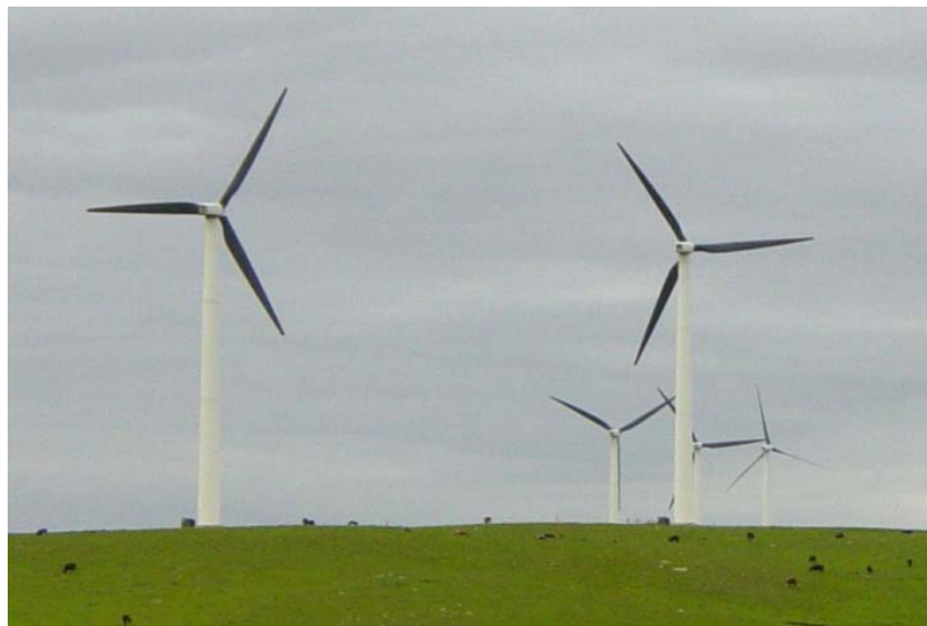
Clean Energy Solution
