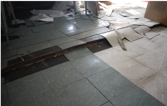
Buckled wood floors in second floor classrooms.
