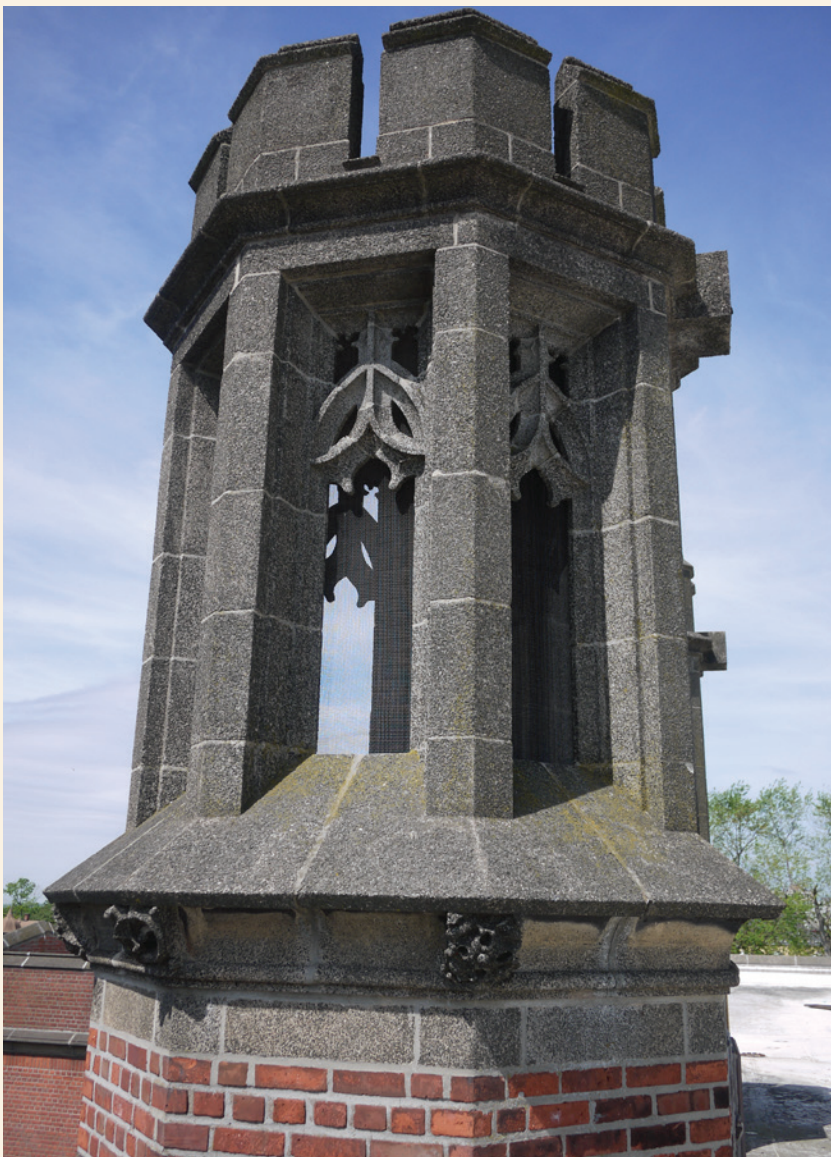
Detail of cast stone turret
