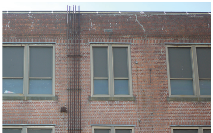
North elevation, showing aging masonry, past repairs to the parapet, and general condition of aluminum windows.
