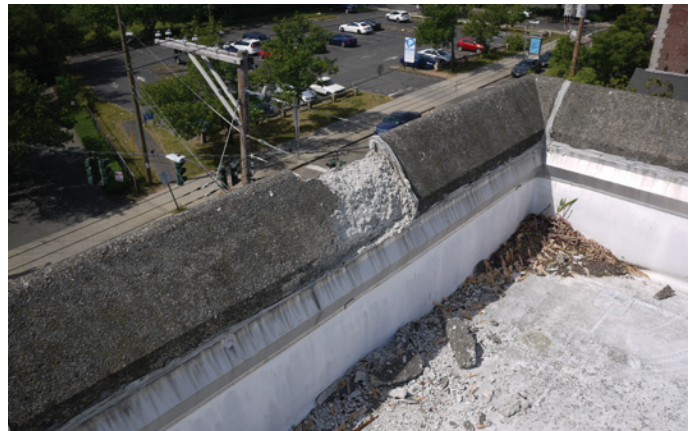
Example of deteriorating stone coping at the southeast corner of the roof.
