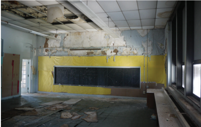
Water damage affecting the ceiling, wall, and floor of a second floor classroom on the northeast corner.
