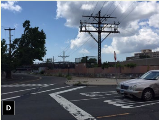
D Union St at Fair St (facing south)
