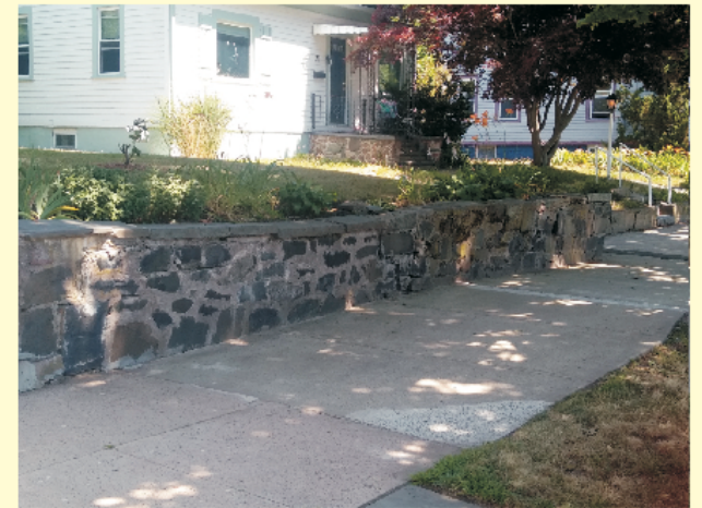
The adjacent stone wall at 81 South Water Street
