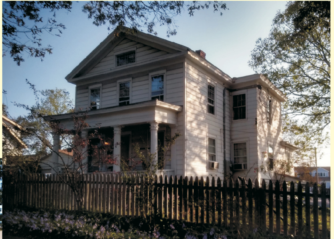
WEST View from Howard Avenue
